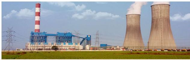
Nabha Power Limited (NPL), a wholly owned subsidiary of L&T Power Development Limited, has set up and operating a 2x700 MW coal based Supercritical Thermal Power Plant at Rajpura, Punjab.
