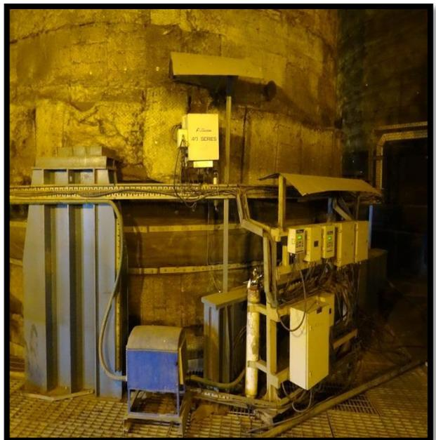
**Pic-2 Continuous emission monitoring system installed at main stack for measurement of Particulate Matter & Gaseous Emissions.**
