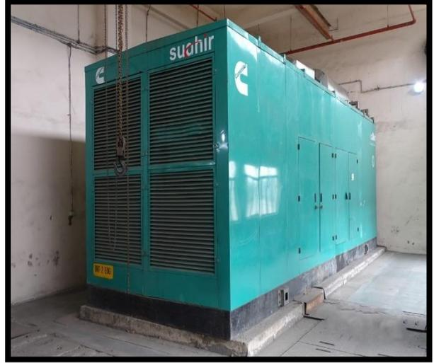
**Pic-2 Acoustic enclosure provided at Diesel Generator.**
