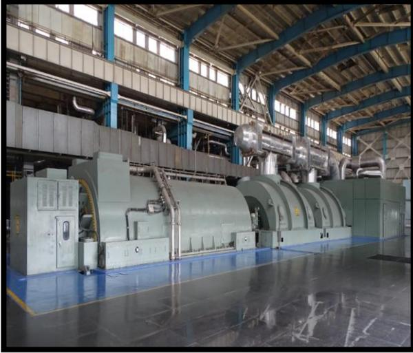
**Pic-1 Acoustic enclosure provided at Turbine Generator.**
